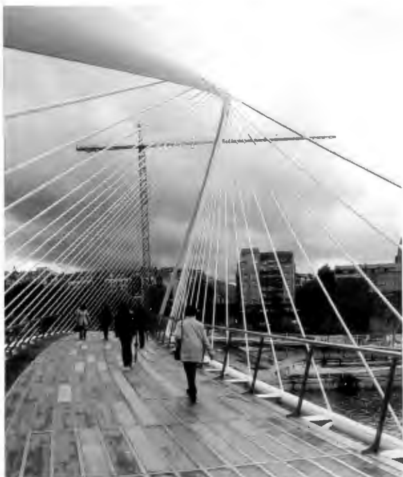
Pasarela Zubi Zuri over Ría de Bilbao (left) and Bilbao's Museo Guggenheim (above).
