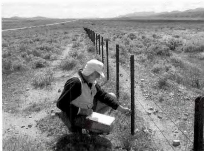
John Pickard inspects the massively over-engineered (but still stock-proof!) fence built for the railway north of Hawker, SA in the 1890s.
