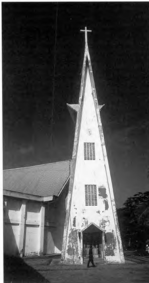
Above: East Timorese church, damaged but still standing. Left: View from wrecked Governor's house on the road to Dare.
